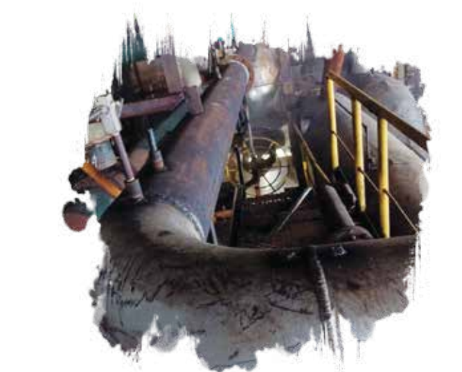
Transfer of Bryant Evap exhaust supply to High Side exhaust line to address blow-off issue.
