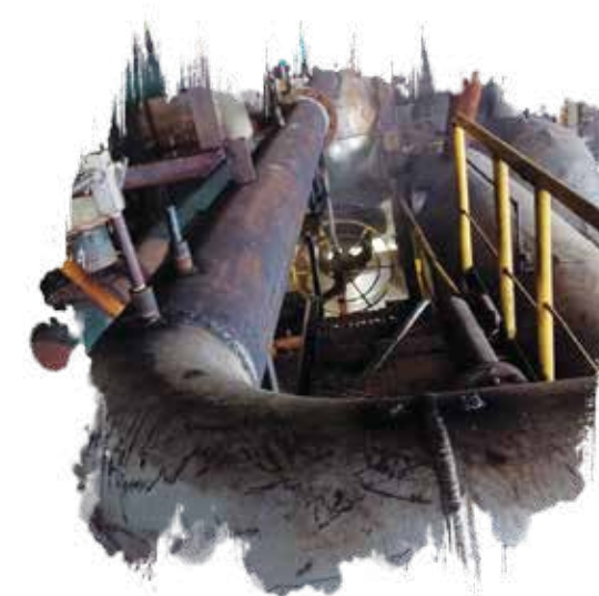
Transfer of Bryant Evap exhaust supply to High Side exhaust line to address blow-off issue.
